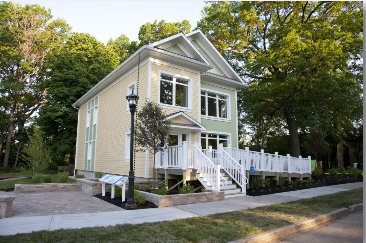
PNC SmartHome at the Cleveland Museum of Natural History in 2011, the first building in Ohio to earn Passive House certification for energy performance. How can communities promote more green building and preservation of historic buildings?
